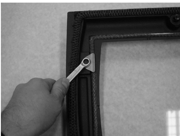
Fig. 11. Tightening The Glass Clip
