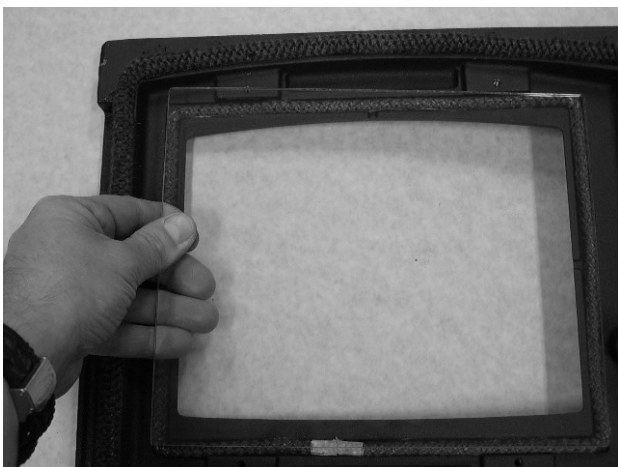
Fig. 10. Positioning The Glass
