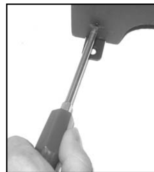
Fig. 5 Inserting and tightening the screws.
